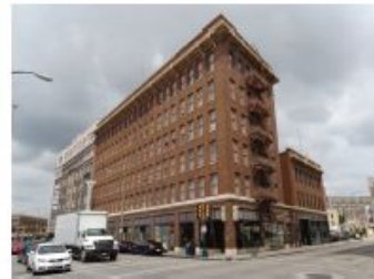
Calcasieu Building on Broadway
