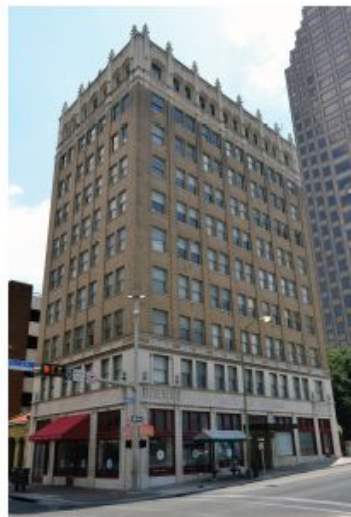
Exchange Building on E. Pecan St.
