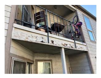
Signs of possible water or termite damage.
