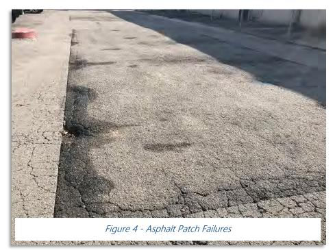
Figure 4 – Patch failures are also a distortion pavement failure. As shown in Figure 4, asphalt patches are present throughout the community and all of them present distress in their outmost layer. Asphalt patches deteriorate at a rate influenced by compaction, material selection and the quality of the surrounding or underlying pavement structure.
