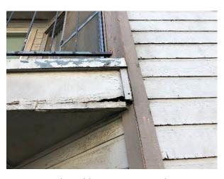
Signs of possible water or termite damage.
