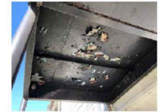
Rotted steel sheet on bottom of stair landing.
