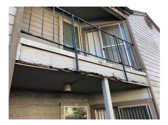
Signs of possible water or termite damage.
