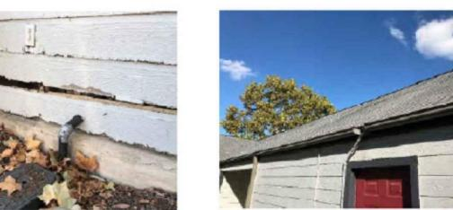
Waviness of roof decking. Signs of possible termite or water damage.
