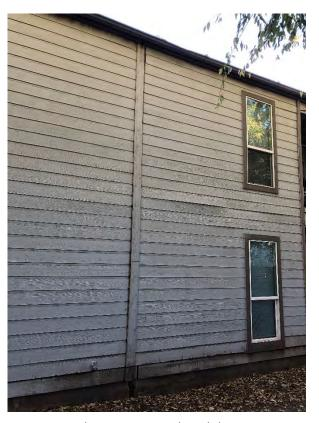
Rigid expansion joint board showing signs of movement.
