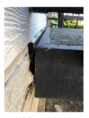
Stair landing connection integrity loss.
