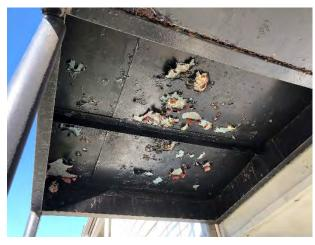
Rotted steel sheet on bottom of stair landing.
