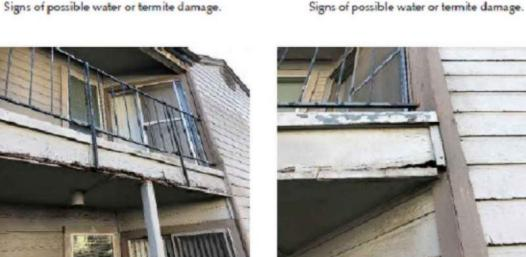
Signs of possible water or termite damage. Signs of possible water or termite damage.
