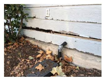
Signs of possible termite or water damage.
