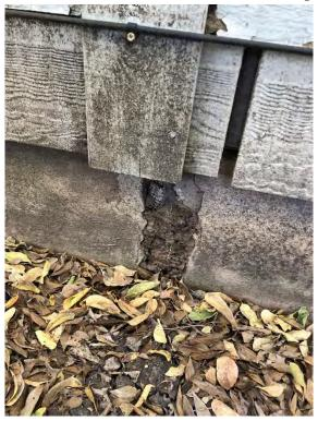
Base of rigid expansion joint showing signs of movement.
