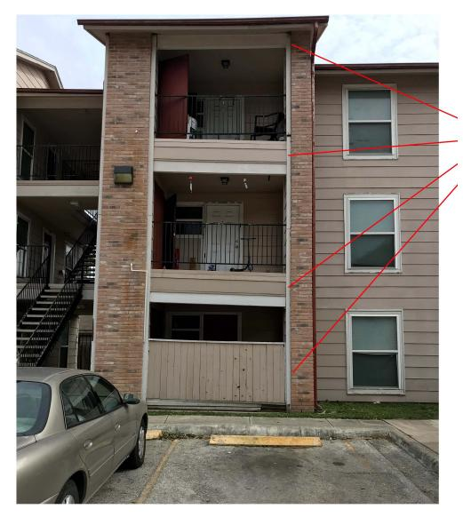
Floor joist, decking, top/ bottom plates, and any other damaged elements , e.g. railing, siding, soffit etc. need to be replaced.
