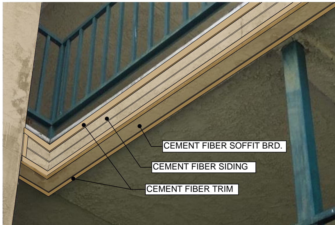
VIEW OF CORRIDOR EDGE AFTER REPAIRS
