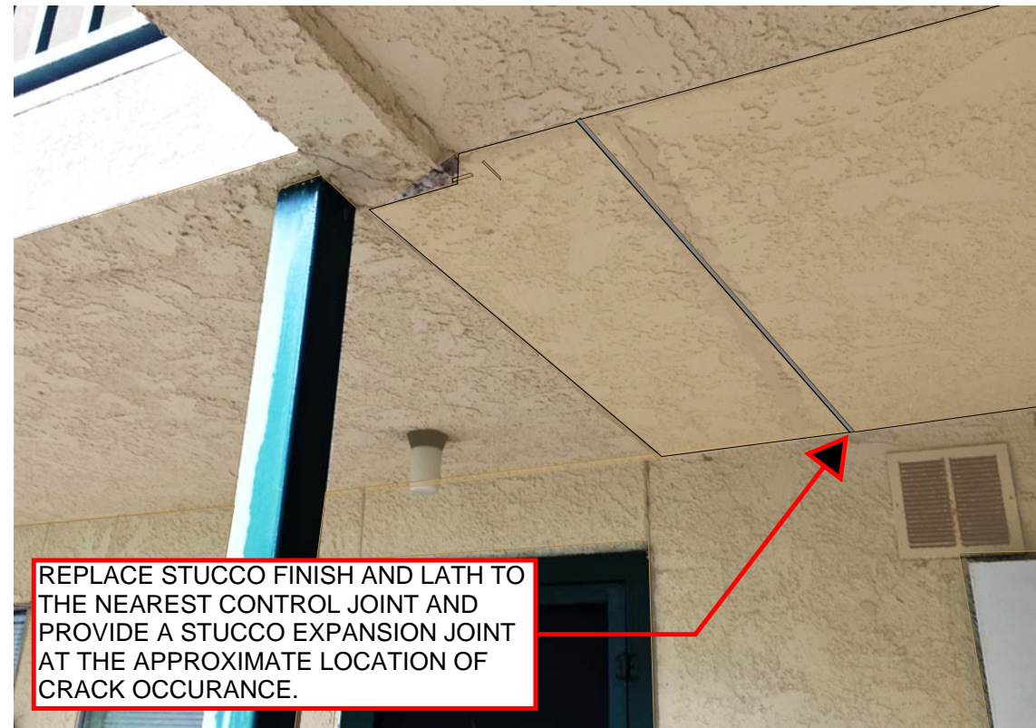
VIEW OF CORRIDOR EDGE AFTER REPAIRS
